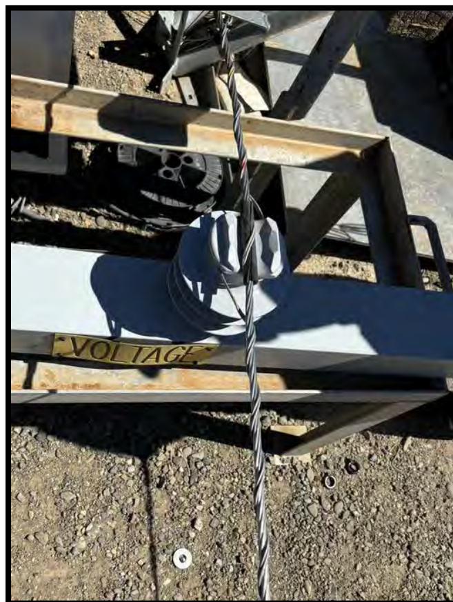
Figure 5. Fastening Method: F-neck
