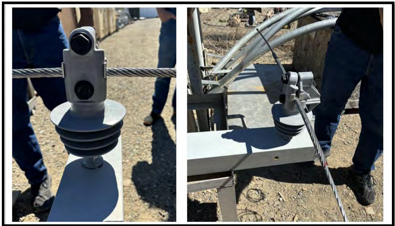
Figure 6. Hand Tie and Preformed F-Neck Connection Prior to Installation
