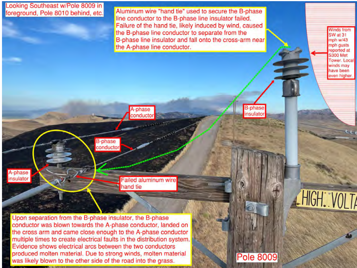
Figure 11. Condition of Pole 8009 on June 1, 2024, after the Fire Initiated (A- and B-phase lines in close proximity)
