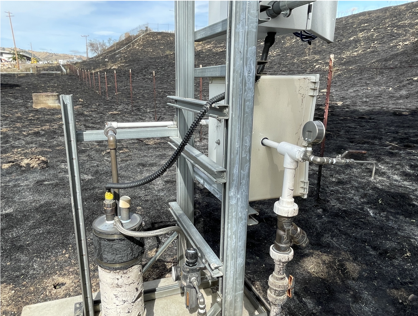
CGSA GWTS extraction well W-7P. Significant damage.
