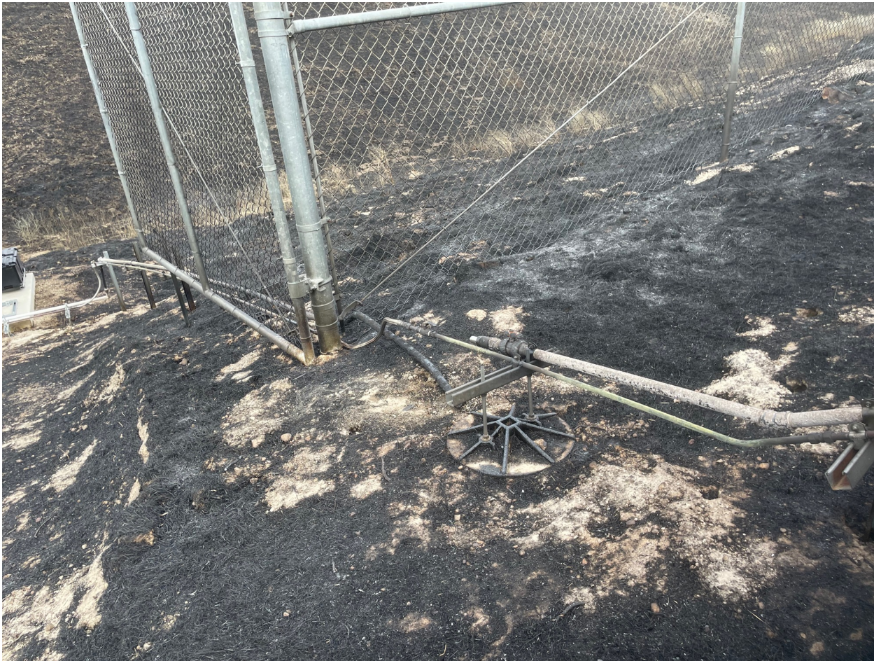
832-SRC GWTS pipeline.
