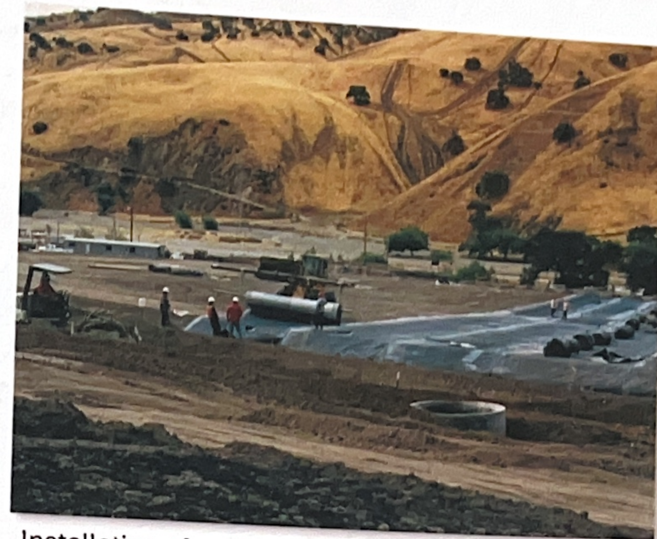
Installation of engineered cap at the Pit 6 Landfill
